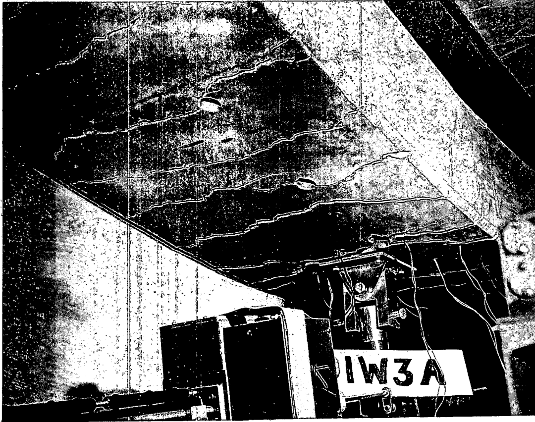
Fig. 5—Photograph showing tension cracks beneath slab IW3A.
